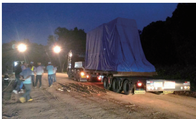
Figure 2: Arrival of Module No. 1 Transporting at night to secure work hours during the day
