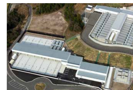
Opened Matsue Data Center Park (2011)
