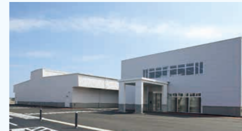
Matsue Data Center Park (Matsue DCP) Shiroi Data Center Campus (Shiroi DCC)
