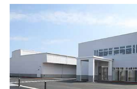
Opened Shiroi Data Center Campus (2019)
